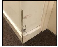
Walls gouged, wallpaper torn and hanging, and corners of walls and door frames battered, are just some examples of regular damage to communal areas.
